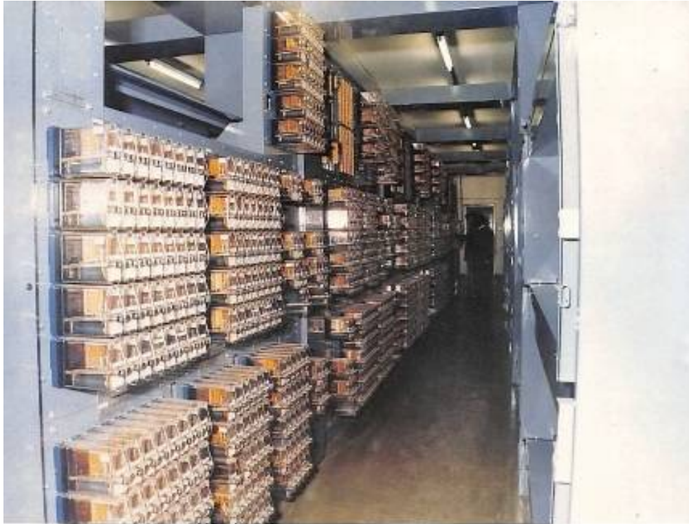
Figure 198 - Westinghouse Westpac MkIVA geographical interlocking, Bedford. © Siemens.
