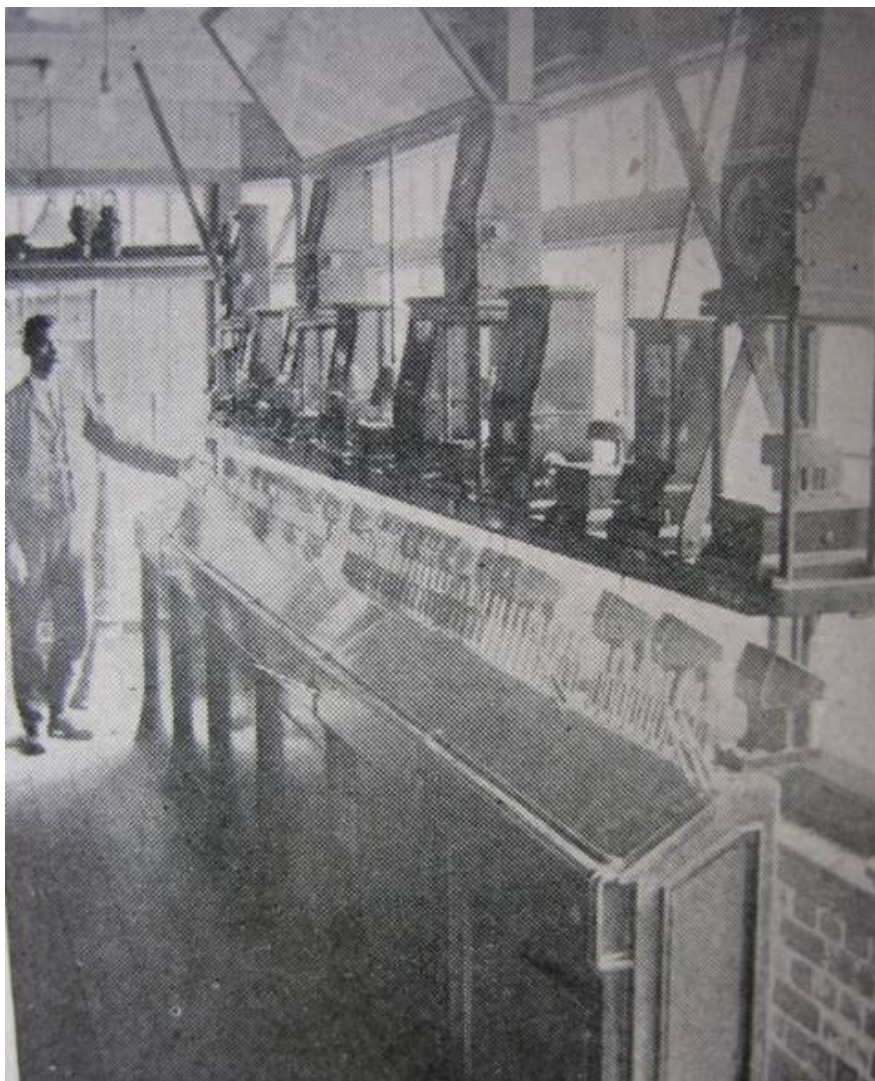
Figure 172 - Siemens All-Electric PF(L), Snow Hill North.
