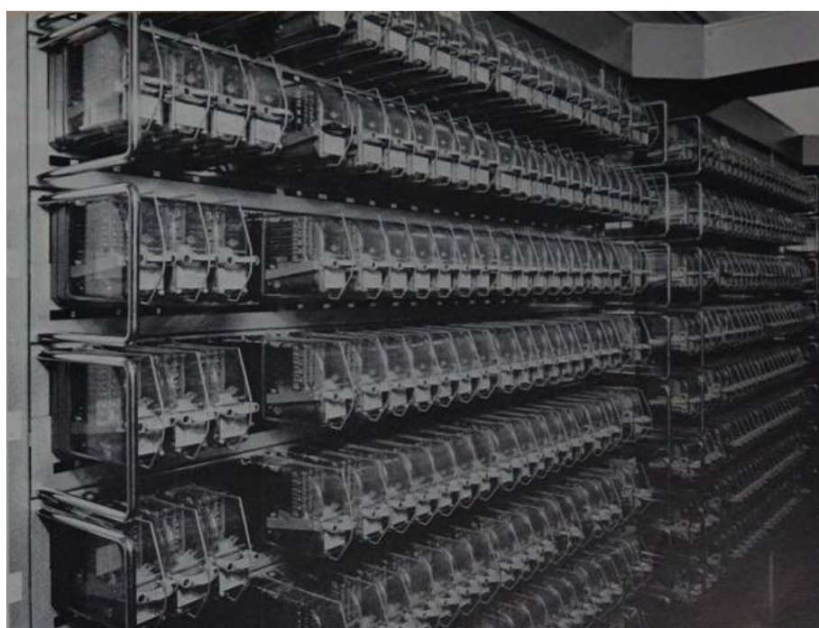
Figure 189 - SGE geographical interlocking, Paddock Wood. © Alstom.
