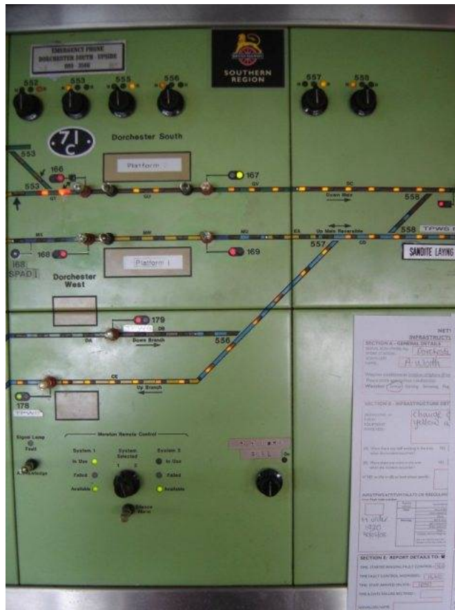
Figure 152 - Westinghouse M5 NX(PP)[+], Dorchester. © Network Rail
