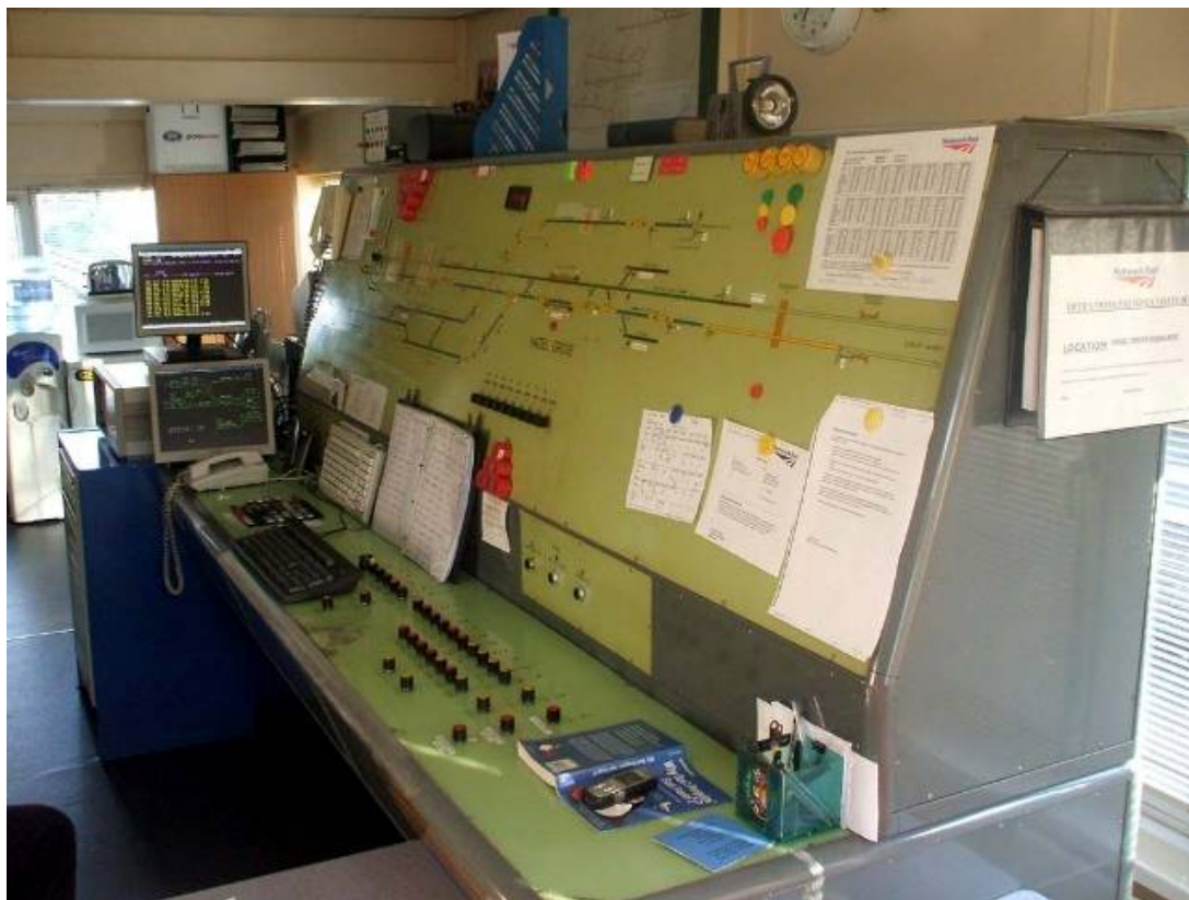
Figure 29 - BR(LMR) OCS[+], Hazel Grove (with replacement fascia). © Stephen Lawton
