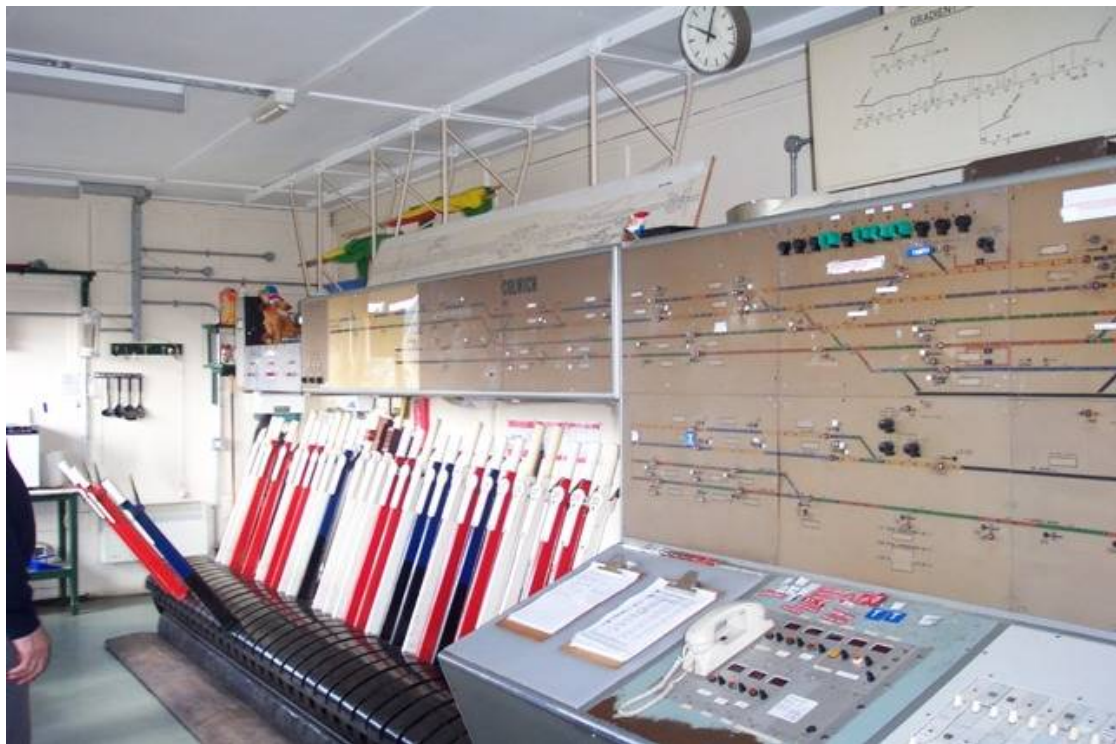
Figure 33 - BR(LMR) Frame / NX(PP)[+] Hybrid, Colwich. © Graham Floyd
