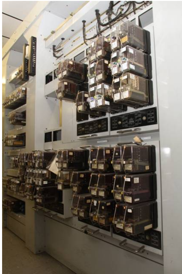
Figure 187 - GEC-GS geographical interlocking, Stewarts Lane. © Simon Foster.
