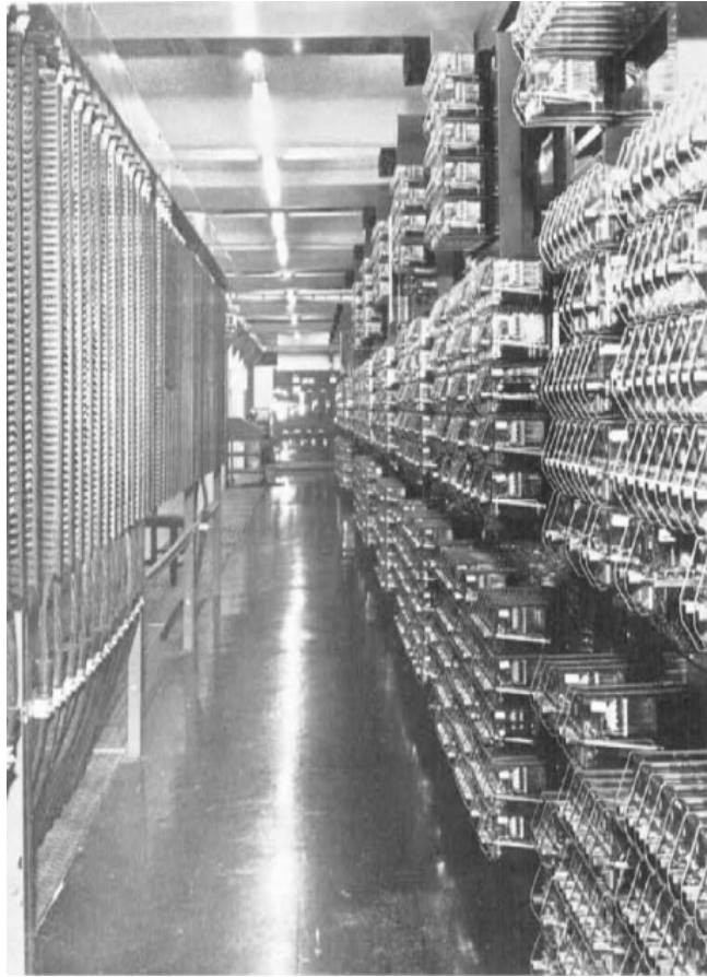
Figure 196 - Westinghouse Westpac MkIIIA geographical interlocking, Warrington. © Siemens.
