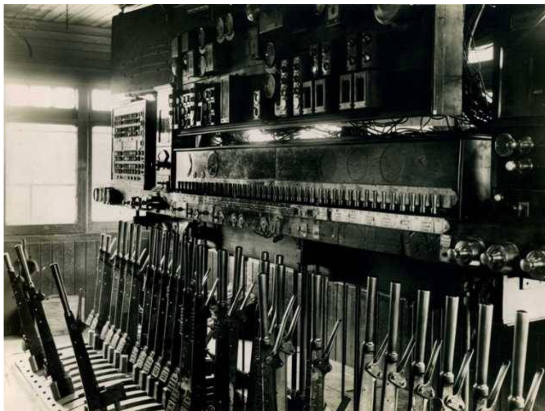
Figure 177 - W R Sykes Frame / PF(S) Hybrid, Port Eglinton. © British Rail
