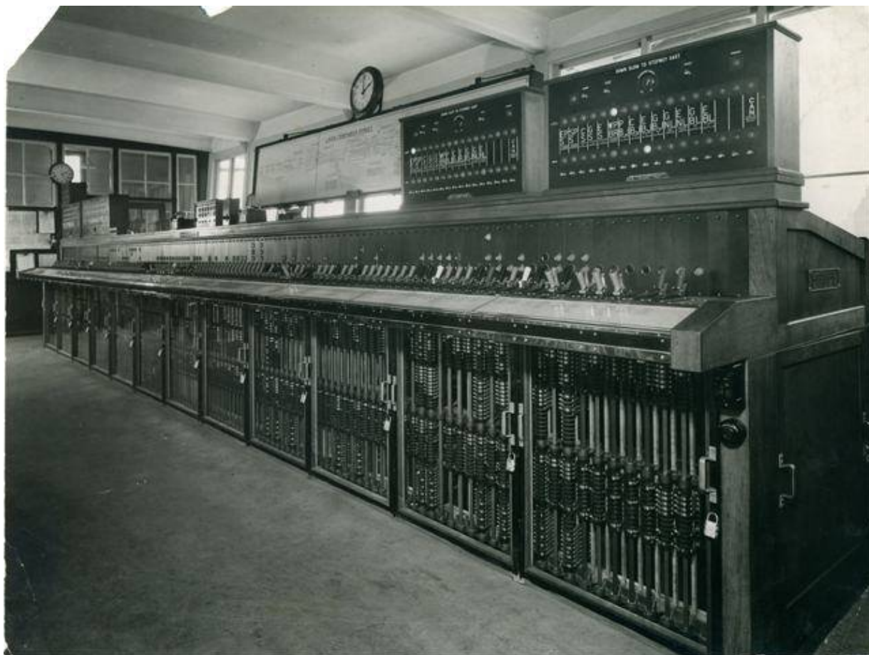
Figure 174 - SGE All-Electric PF(L), Fenchurch Street.
