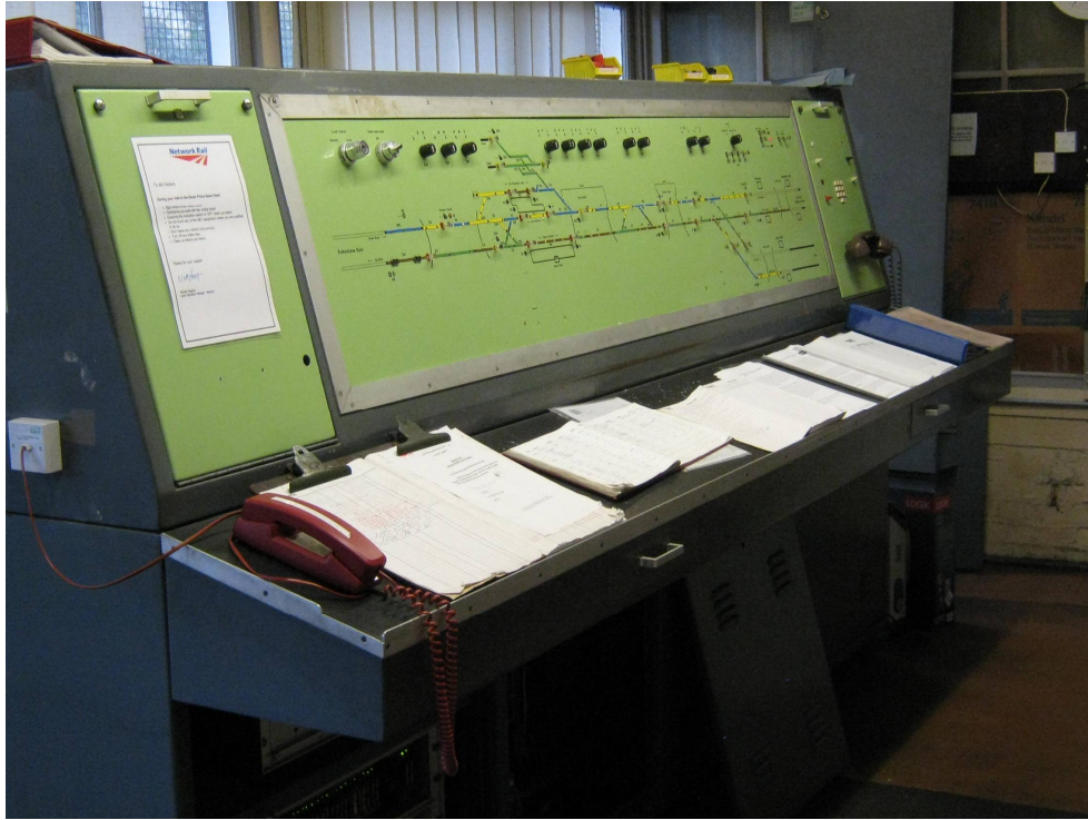
Figure 64 - GEC-GS NX(PP)[+], Dover Priory LCP. © Nick Wellington
