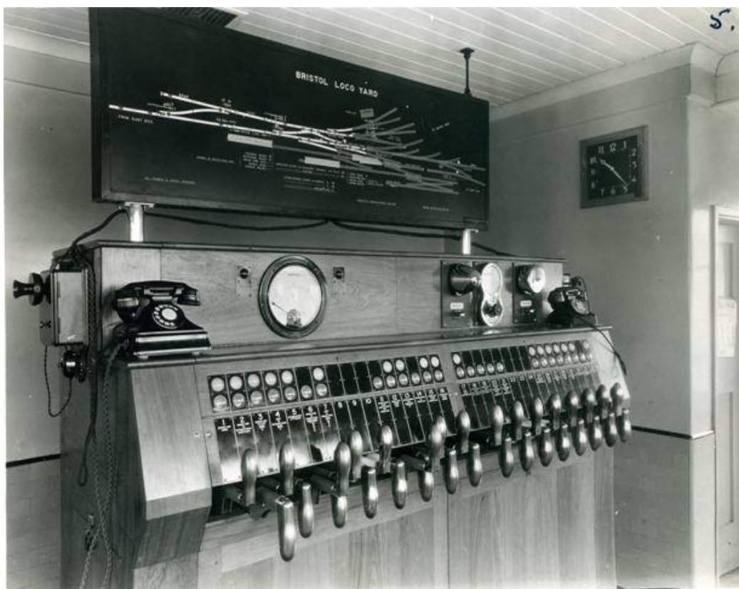
Figure 165 - GRS Type D PF(S), Bristol Locomotive Yard. © F Bromhead (Andrew K Overton Collection)
