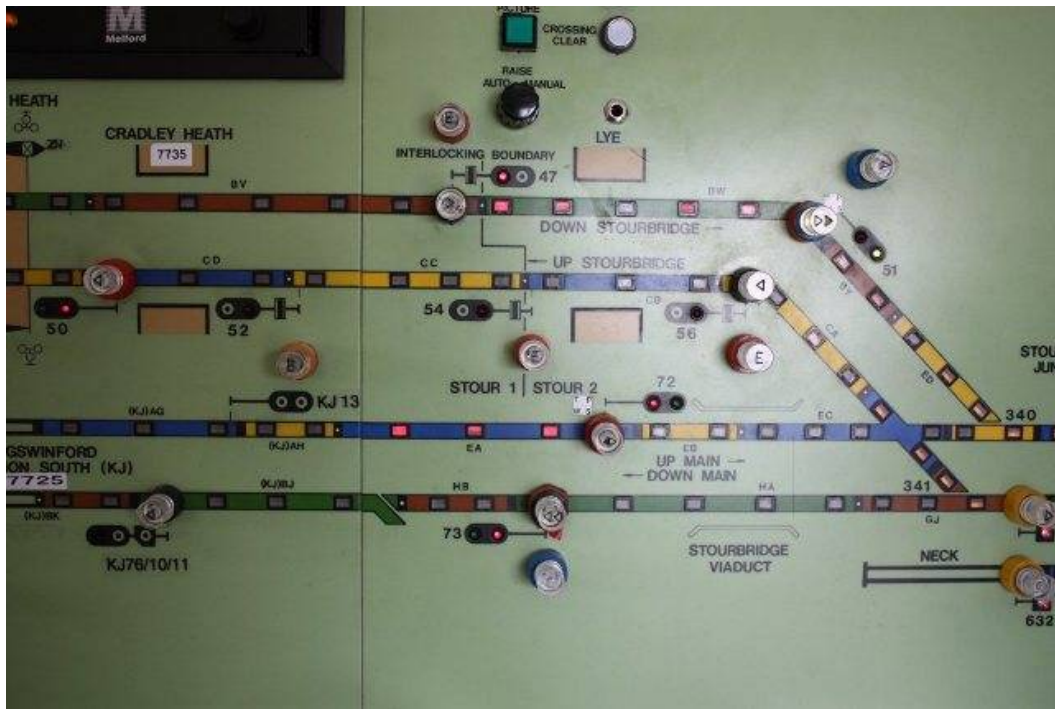
Figure 158 - Westinghouse M4 NX(PP)[+], Stourbridge Jcn. © Danny Scroggins
